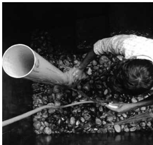
Clean recharge bore and filter material
