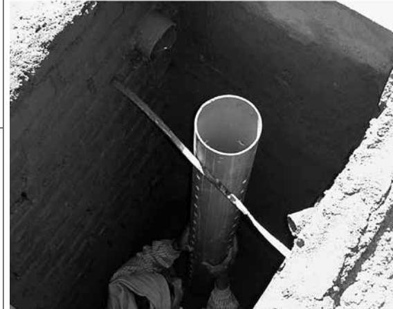
Casing of tubewell (top), slotted pipe (below)
