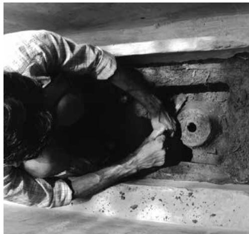
Remove silt from recharge bore
