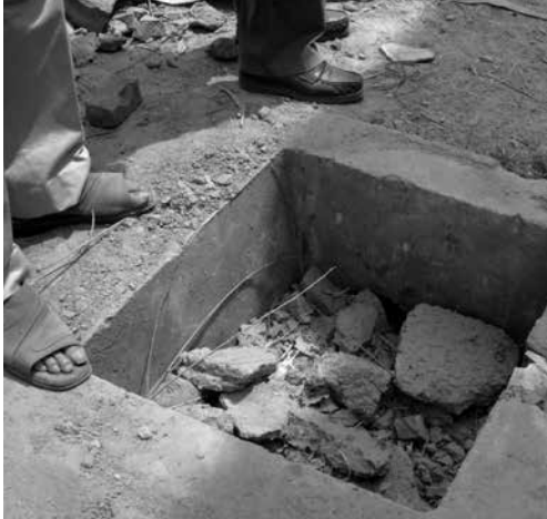
Settlement chamber filled with debris (malba)
