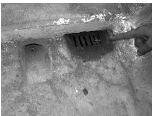
First flush: The left outlet is plugged with cloth during the initial rains. The first flush of rainwater flows into the other outlet which leads into a stormwater drain outside the house. Water is later diverted into the tanka
