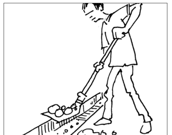
The trench has to be free of debris
