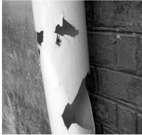
Cracked downtake pipe
