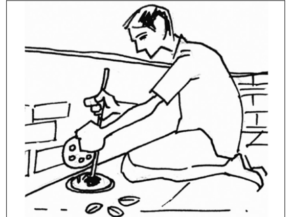
Keep the outlets clean
