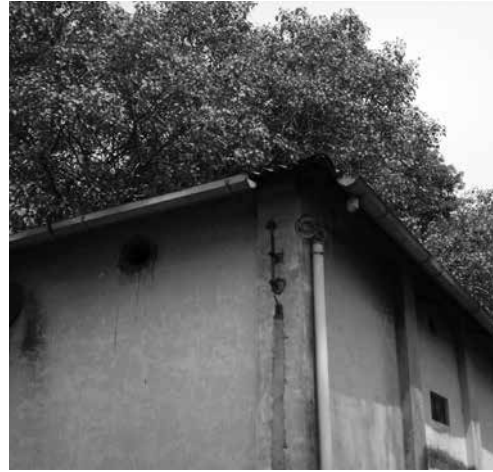
Downtake pipe not connected to the roof
