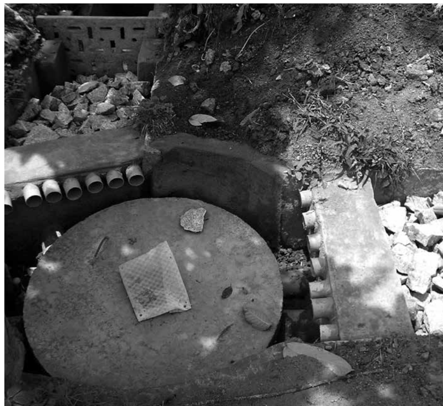
A recharge well in a stormwater drain. The jelly stones desilt the water before it enters the well
