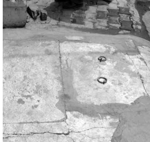
Cracked RCC cover of a recharge well
