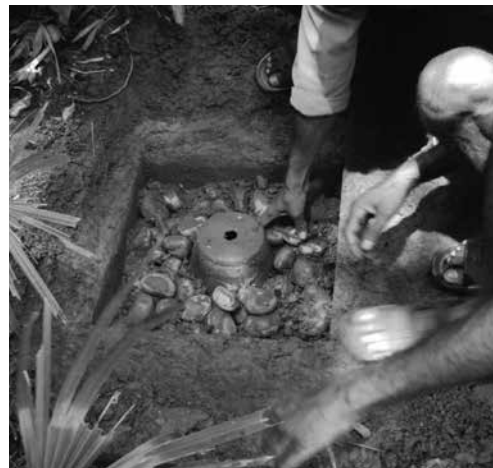
Remove filter material (pebbles) from pit
