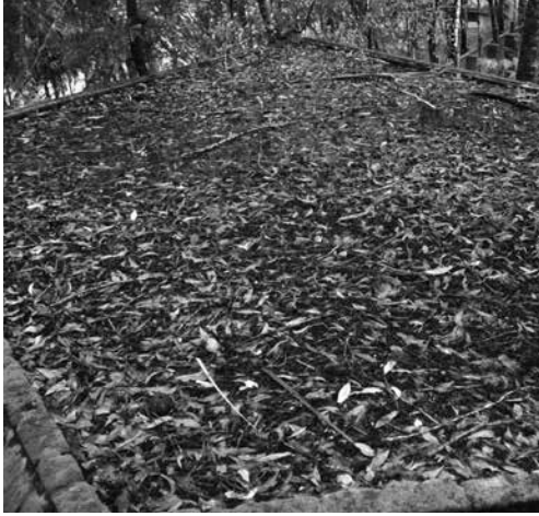
Rooftop covered over by leaves
