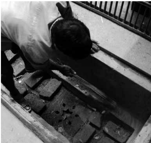
Remove parts of recharge trench for cleaning
