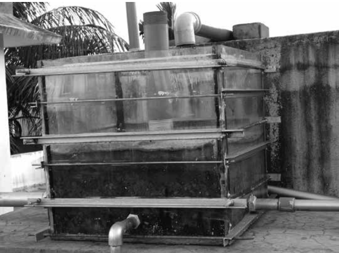
Type of simple sand filter being used in the Association of Engineers building, Kolkata. It has gravel and pebbles
